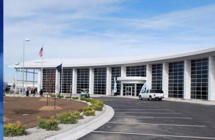
Siemens Wind Turbine Facility, Hutchinson, KS
